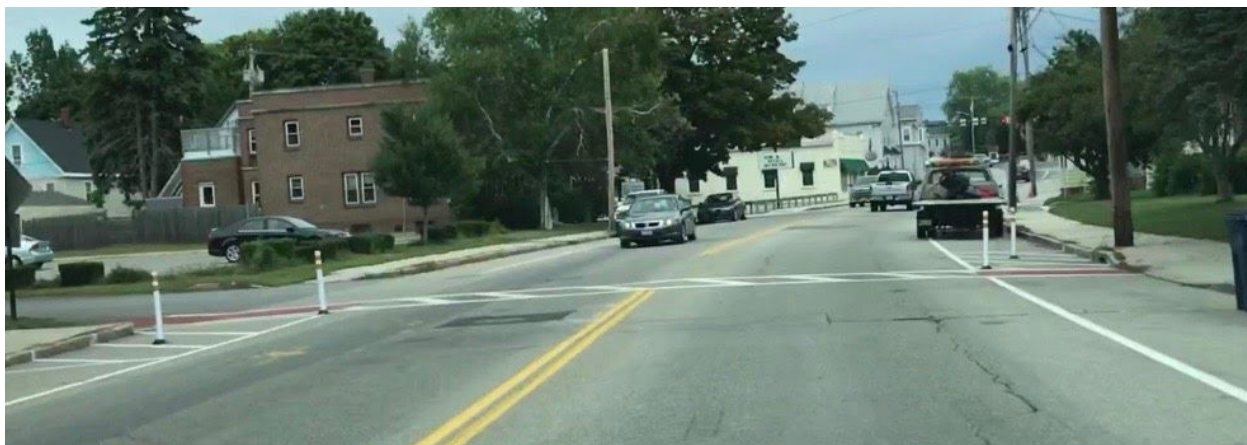
Figure 9: Crosswalk gateway at the Riverside Park access road.
