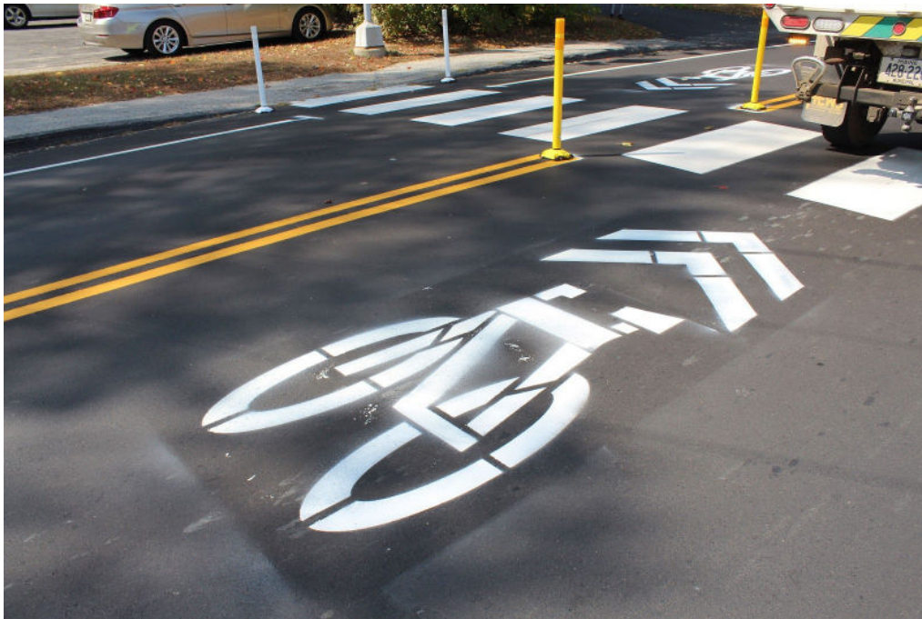
Figure 6: Crosswalk delineator gateway also showing SLM
