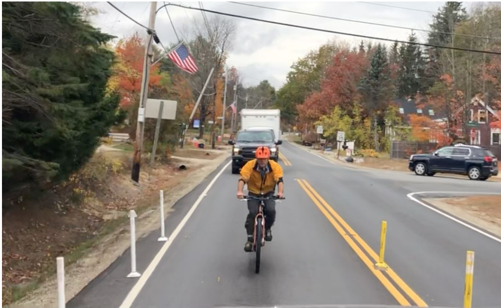
Figure 5: Northern delineator gateway with bicycle rider
